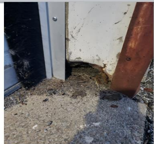
Top Right: Deterioration along overhead doors which leads to rodent infestation
